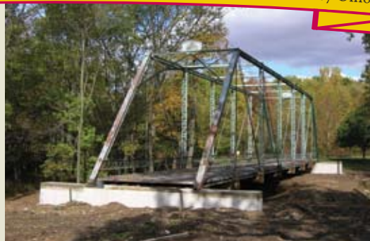
TR 241 Bridge relocated to new location in Riverbend Park
