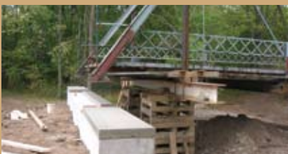
New abutments, new home
